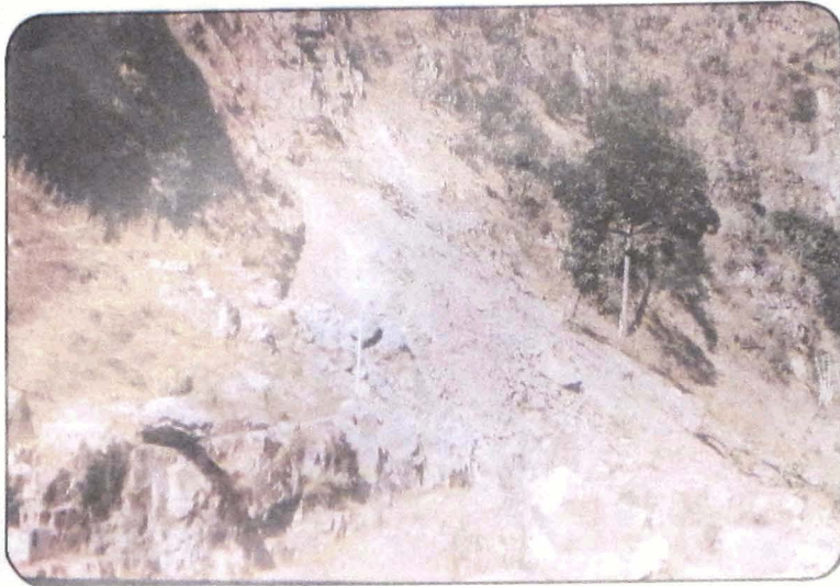
Photo 1 Rock fall cum debris slide initiated in quartzites upslope of the road about a km before Maneri. Note uprooting of a telephone pole in the toe portion of the slide.
