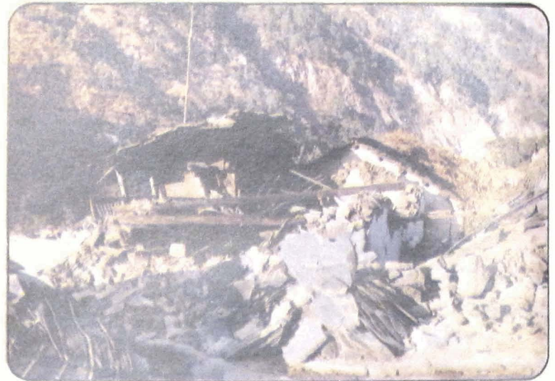
Photo 53 Collapsed and precariously tilted house in Dedsari village.
