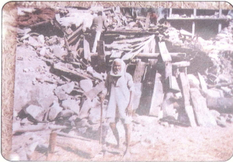
Photo 47 Villagers salvaging roofing timbers from collapsed houses in Jamak. Old man standing amongst ruins.
