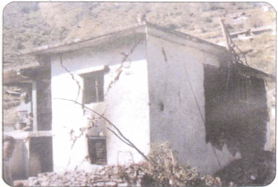
Photo 62 Open shear cracks in NE-SW wall and partial collapse of NW-SE wall in the house of Sahdev Singh of village Pala.
