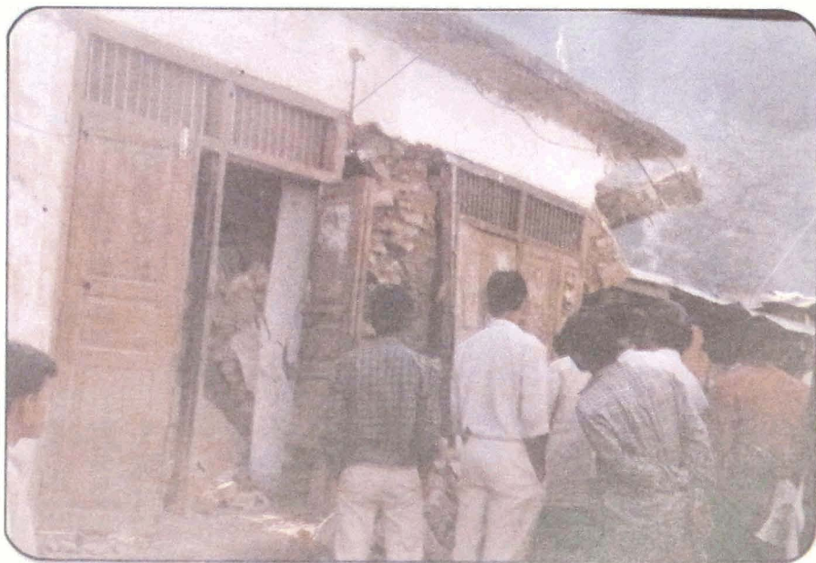
Photo 79 Collapse of shops in Lambgaon market.
