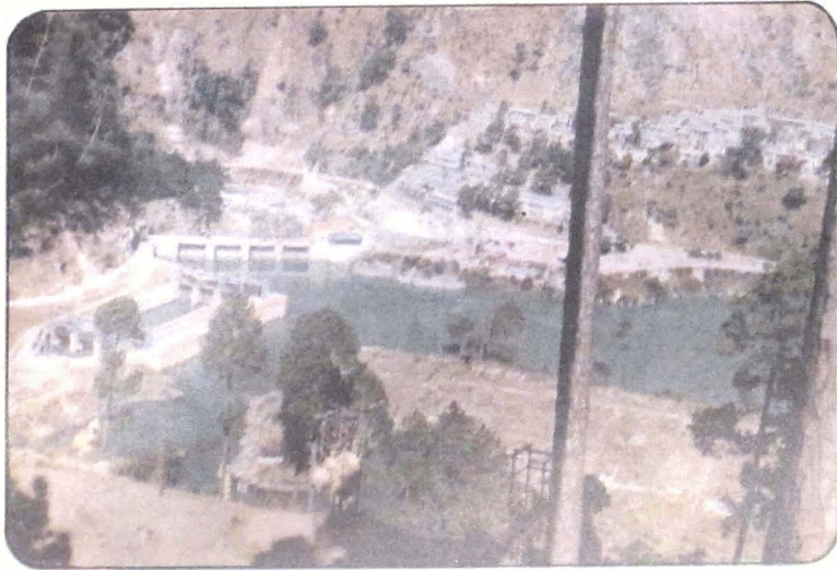
Photo 15 View showing Maneri dam and the appurtenances facing downstream. Maneri colony in the background.
