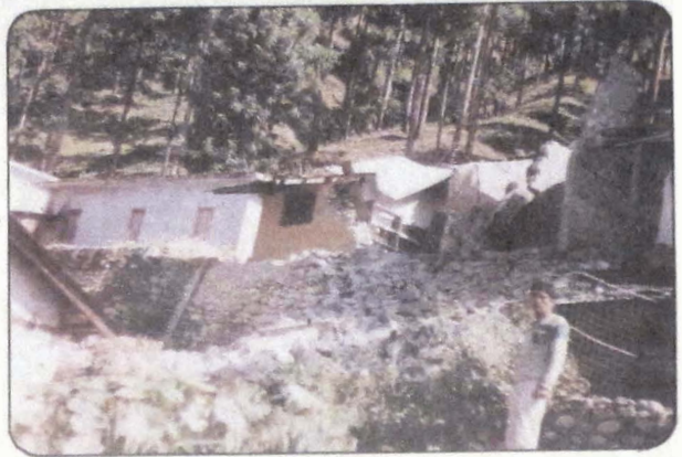
Photo 88 Damage to cluster of houses in Gangani village.
