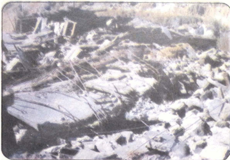
Photo 53 A Complete collapse of type A houses in Dedsari village. RCC roof slab damaged because of wall collapses in one of the houses.
