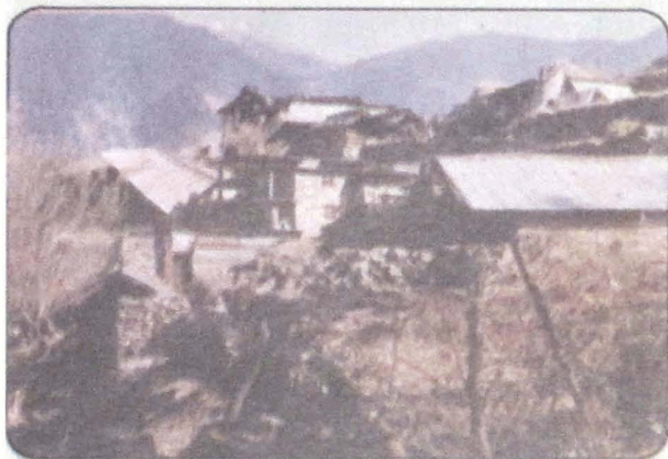
Photo 56 A distant view of damages in Raithal village.
