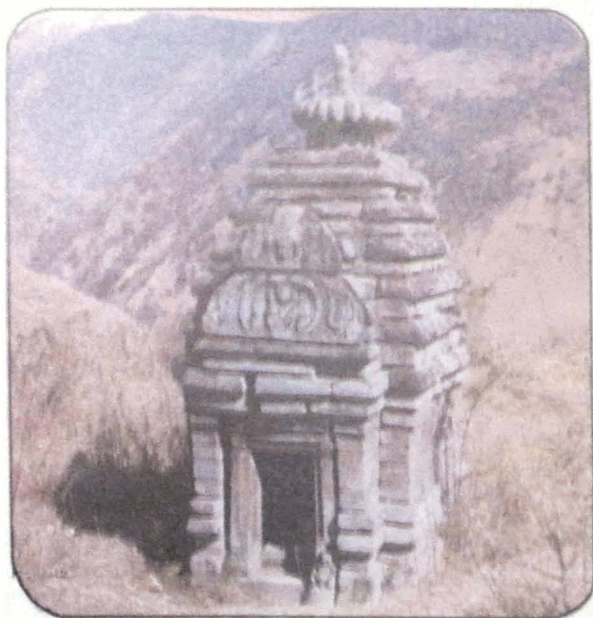
Photo 57 A Old temple near Raithal village, displaying shifting of top cupola (kalash).
