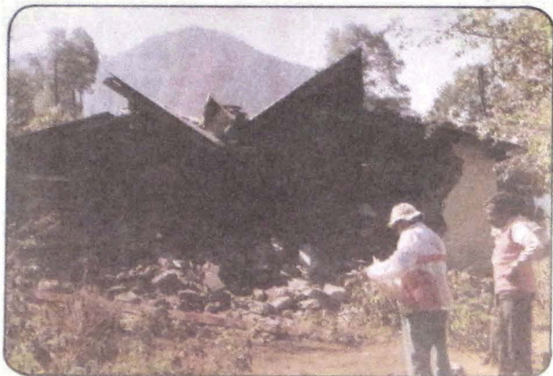
Photo 92 Caving in of the roof of a conventional construction because of partial collapse of supporting walls, Gangani village.
