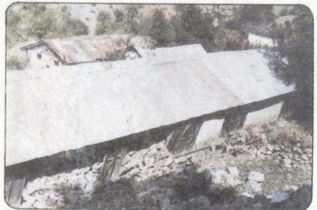
Photo 91 Tilting of the eastern long wall of a conventional house in Gangani village.
