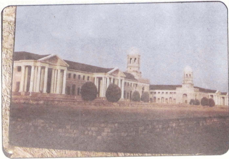
Photo 95 A general view of FRI building, Dehradun.
