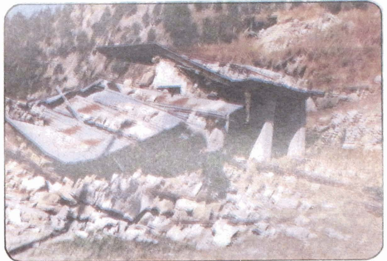
Photo 50 Complete collapse of Kamar school building made of mud masonry with GI sheet roofings.
