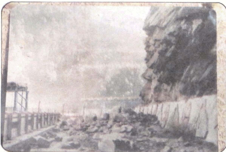
Photo 3 Rock fall in blocky quartzites. Note large rock blocks lying on the approach road to intake structure of the Maneri dam.
